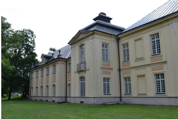
Figure 6 The northern site of the Palace
